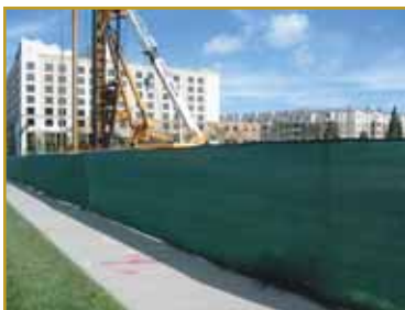
CONSTRUCTION FENCE SCREEN
